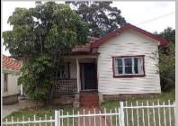
The condition of the walls is generally poor. The external wall timbers show signs of age and weathering. Maintenance and/or repairs will be required. Paint deterioration was present to external surfaces. Maintenance and/or repairs will be required. Severe wet rot decay is present to external walls. Recommend decayed timbers be replaced.
