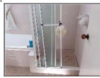
The shower recess was tested and there was no visible water penetration to surrounding areas. IMPORTANT NOTE: This test may not reveal water leaks until the shower is put into constant use and surrounding areas monitored over a period of time. Corrosion/Damage noted at the tap area. Shower screen doors require adjustment, maintenance or repair to operate smoothly.
