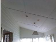
The condition of the ceilings is generally fair. Minor settlement cracks were noted and these are typical of this type of material. Periodic maintenance may be required. Minor cracking is present to cornices. This will require maintenance. Painting is of a poor standard and requires rectification. Peeling paint was noted to ceilings. Repairs are required to ceiling linings.
